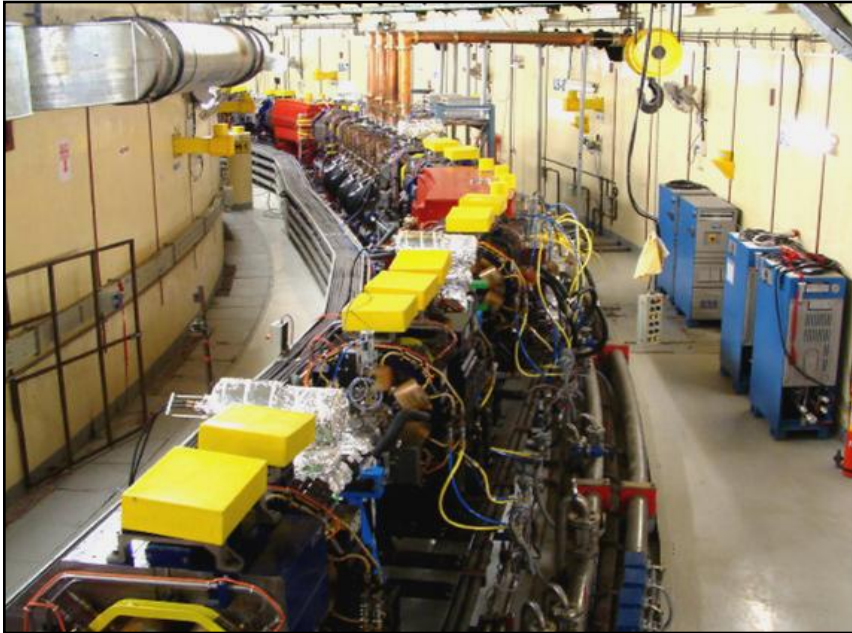
A section of Indus-2 tunnel (172 m)
