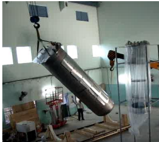
Installation of Cryostat in pit
