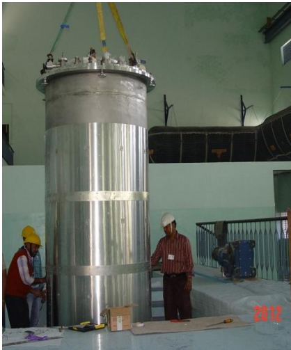
Assembly of external shield
