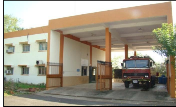
Fire Station operates round the clock
