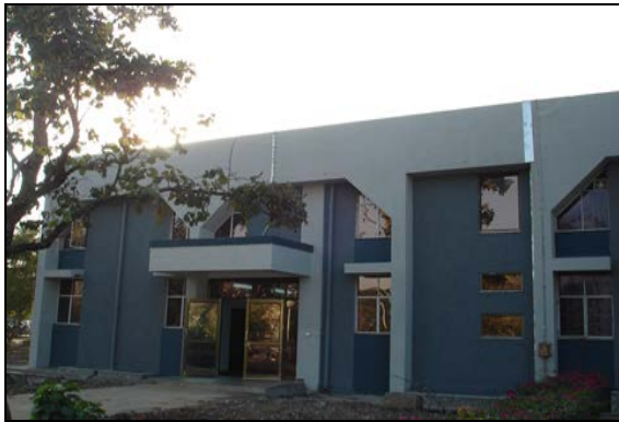
Fig. 66 : Petawatt laser laboratory building.
