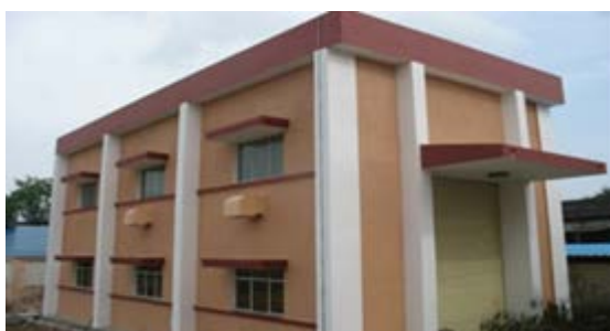
Fig. VII.2.1.1: Ion exchange building.
