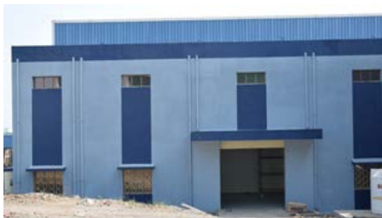
Fig. VII.2.1.3: Support building for clean room of SCRFL laboratory.
