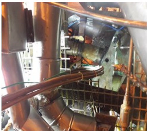
Fig. IV.4 :Remote laser cutting of double check valve pipelines at four different locations of KKNPP-1 reactor at Kudankulam.
