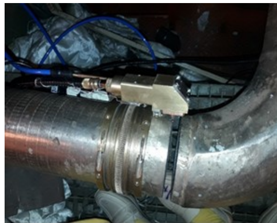
Fig. IV.4 :Remote laser cutting of double check valve pipelines at four different locations of KKNPP-1 reactor at Kudankulam.
