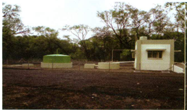
Picture I.2.1: A view of NISARGRUNA Biogas Plant in RRCAT
