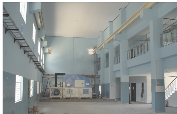
Photograph showing inside view of CPL building
