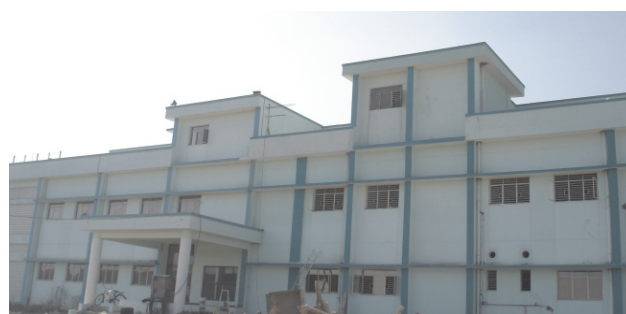
Photograph showing front view of ATF extension
