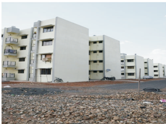
Fig. I.1.1: View of Type I-A houses in CISF Colony
