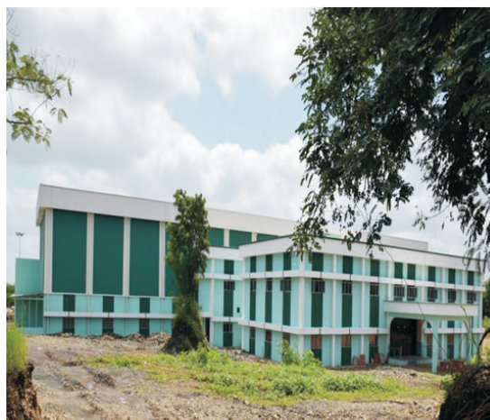
Fig. I.1.3: View of the PEB of Cryomodule Engineering Laboratory
