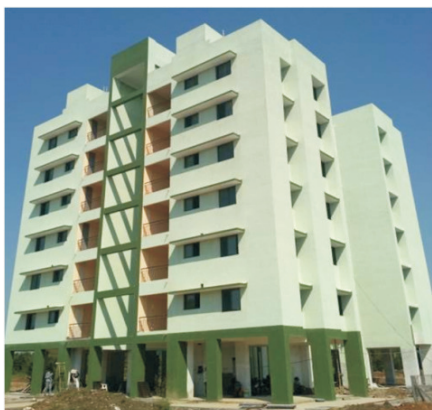
Fig. I.2.1: Photograph of the multistoried type III C Nilgiri Tower.
