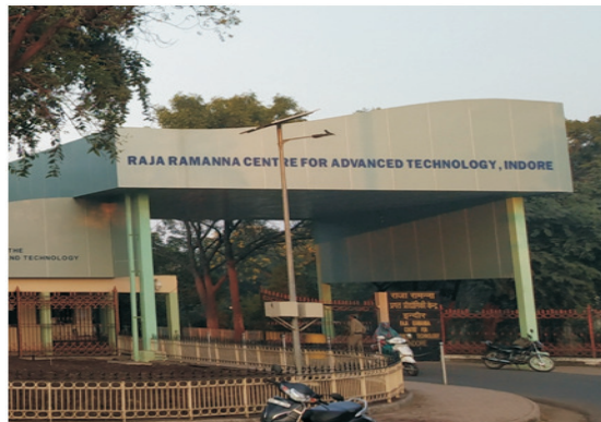
Fig. I.2.3: Photograph of main gate of RRCAT premises.
