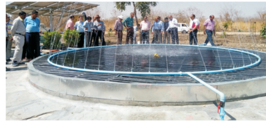
Solar powered pump for horticulture needs.
