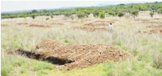
Continuous contour trenching on slopes.
