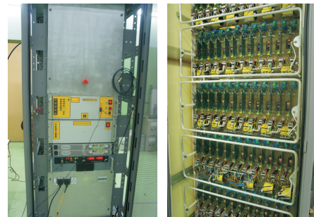
Fig. A.13.3: Photograph showing the front and rear view of the modulator.
