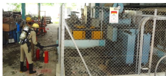
Fire mock drill at UHV transformer unit.
