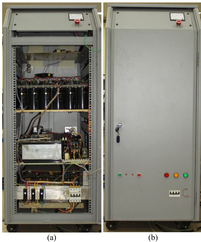
Fig. T.2.2: Photographs of 5 kW power supply for flash lamp pumped 250 W average power pulsed Nd:YAG laser (a) internal front view, and (b) outer front view.
