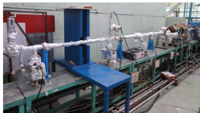
Fig. A.8.1: Photograph of newly installed vacuum system of TL-2 (Indus-1 hall).
