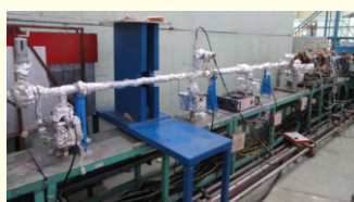
Photograph of newly installed vacuum system of TL-2 (Indus-1 hall).
