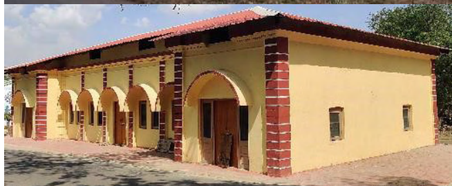
Baggi-khana before (top) and after (below) renovation.
