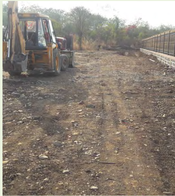
Fig. 23 The debris being removed with the help of JCB (2/2)
